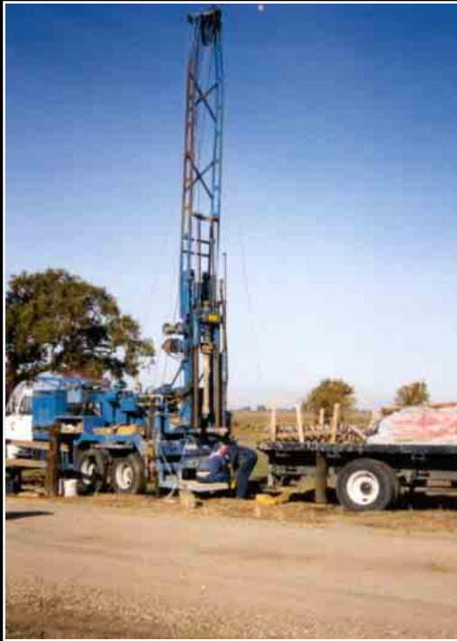
Typical Drilling and Well Construction Activity
