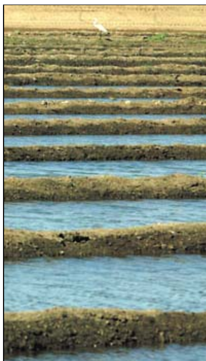
An egret stands among furrows that help promote percolation in recharging the groundwater supply at the Stockton East Water District Water Treatment Plant. (Jennifer M. Howell/News-Sentinel)
